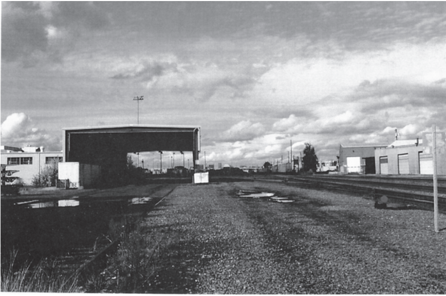
Brooklyn Rail Yard in southeast Portland. Photos by Suzie Boss.
